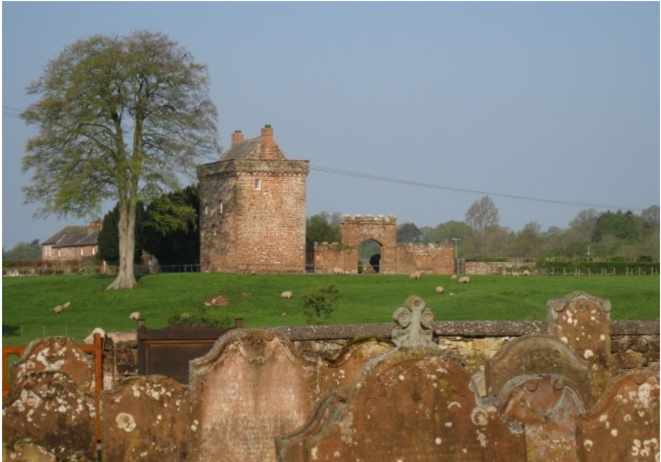
Graham Tower at the new Kirkandrews on the Esk.
